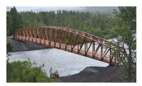
↑ Don't worry, Hess Creek isn't flooding. This bridge is located in Chugach National Forest in Alaska, and at 280 feet is the longest clear-span timber bridge in the U.S. The Hess Creek bridge will look just like it, but will measure 220 feet long. It's scheduled for completion in August 2015.
