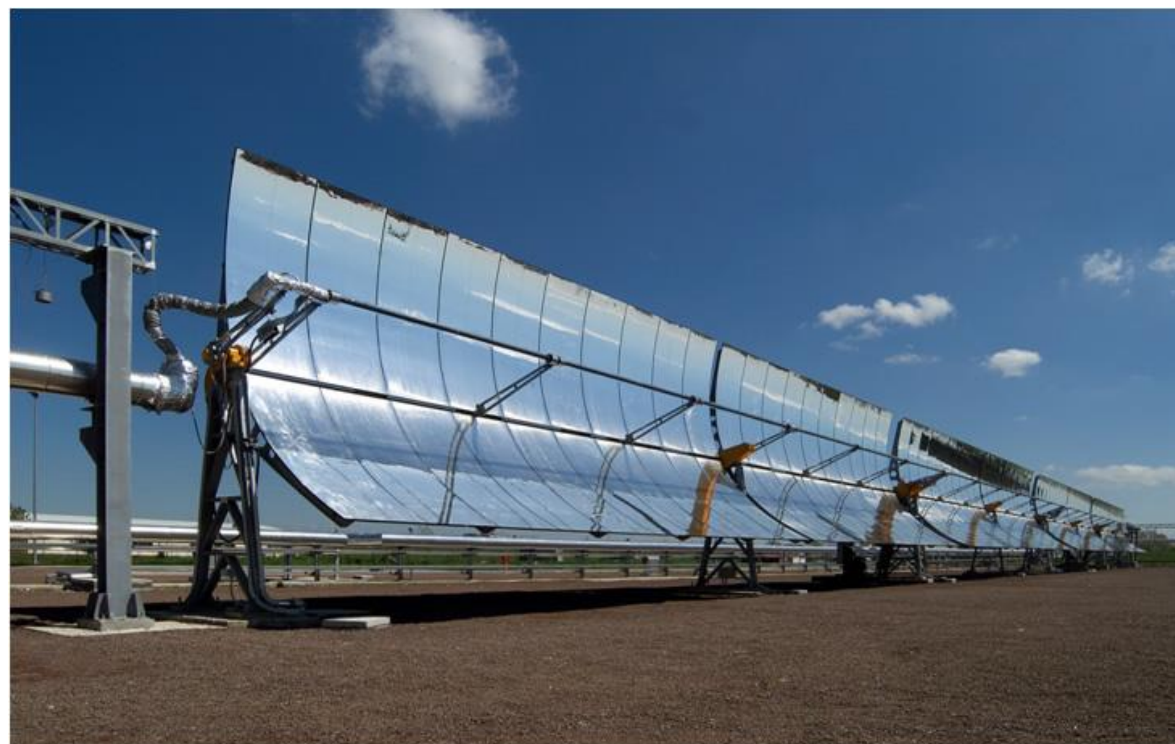
Figure 4. Parabolic troughs on an automated solar tracking system.
