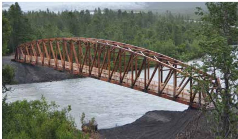
↑ *Don't worry, Hess Creek isn't flooding. This bridge is located in Chugach National Forest in Alaska, and at 280 feet is the longest clear-span timber bridge in the U.S. The Hess Creek bridge will look just like it, but will measure 220 feet long. It's scheduled for completion in August 2015.*
