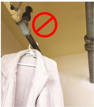
Do NOT hang anything on exposed pipes, sprinkler heads or overhead grilles.
